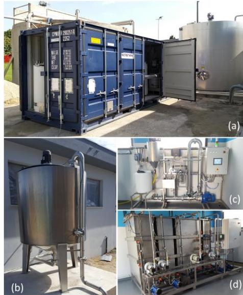
**Figura 8 (a) Rotating Belt Filter for the sieving of wastewater; (b) fermentation unit for the production of VFAs; (c) ceramic membrane for the solid/liquid separation and crystallizer for P-salts production; (d) Units in SBRs-modules for nitritation, PHA storing biomass selection and PHA accumulation.**
